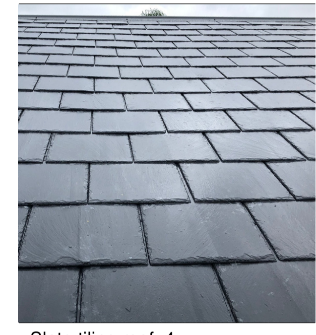
Slate tiling roof_4
